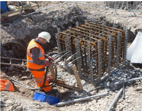
Energy Pile Installation
