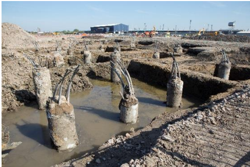
Energy Pile Installation
